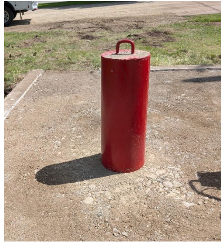
Figure 5: Well 1 Building Removal and Aquifer Protection.
