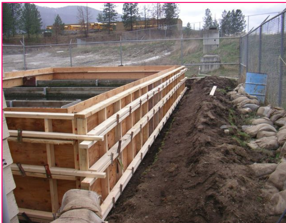
Contact Chamber Wall Extension
