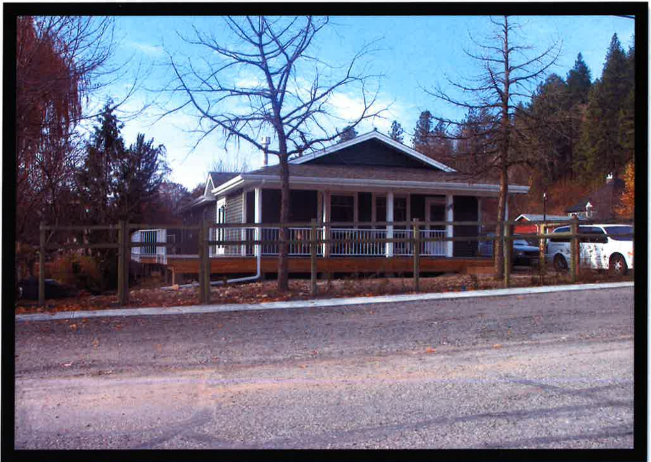
New Modular Home Completed on 3 rd Street
