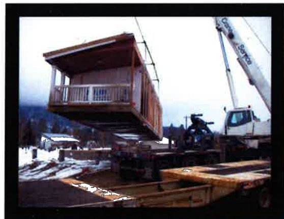
Home being placed on the foundation
