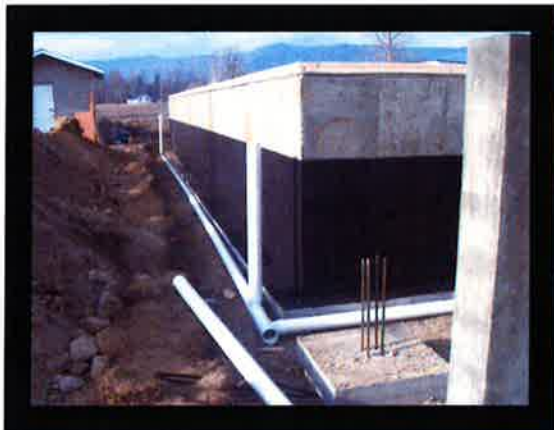
Foundation for a Modular Home
