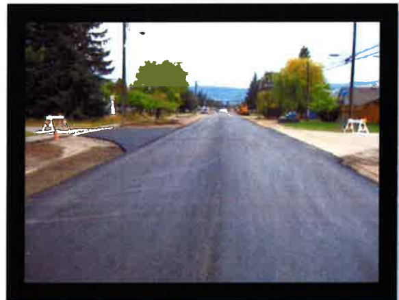
68 th Ave. Paving
