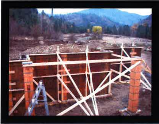
Foundation being prepared
