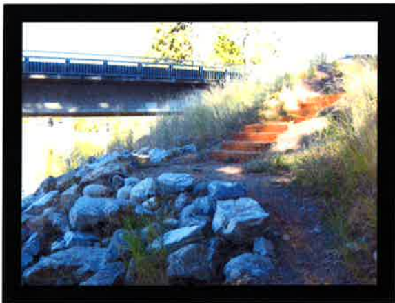
Spragett Bridge Tubing Parking Lot
