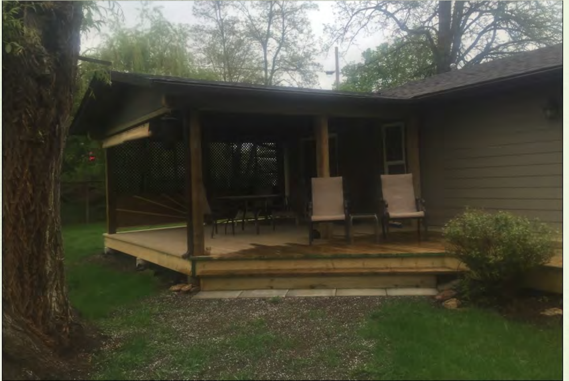
New Outdoor Living Space - Completed on 2nd Street
