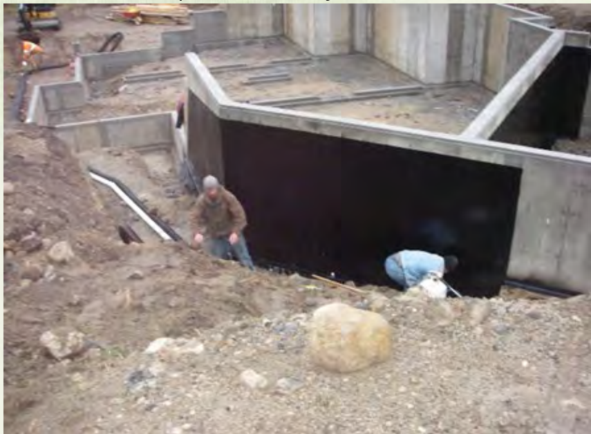
Complex Foundation for New Home
