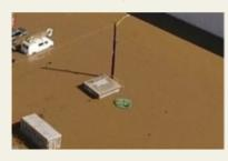
This lift station flooded in 2018. In order to mitigate the risk of future flooding, the building and controls need to be raised. Electrical service may need to be moved, and pumps may be replaced with more efficient units.
