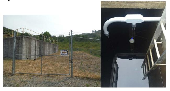
The High Zone Reservoir is a single-celled, ground embedded reservoir, with a depth of 7 m. It is constructed of concrete. The total floor area is  $94 \text{ m}^2$  and it stores  $450 \text{ m}^3$  of potable water.
