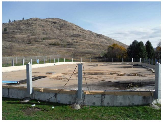
The East Zone Reservoir is a single-celled, ground embedded reservoir, with a depth of 4 m to 4.5 m. It is constructed of concrete with a Hypalon liner and a floating membrane. The total floor area is  $1,300 \text{ m}^2$  and it stores approximately  $4,000\text{m}^3$  of potable water.
