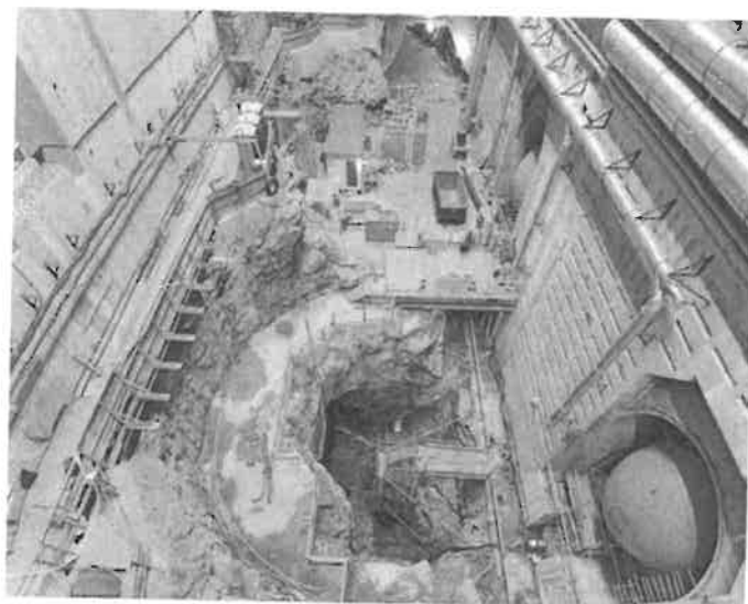
Two empty bays at Mica Generating Station that will house the new 5th and 6th Mica generating units being installed by the Mica Units 5 and 6 Project.
