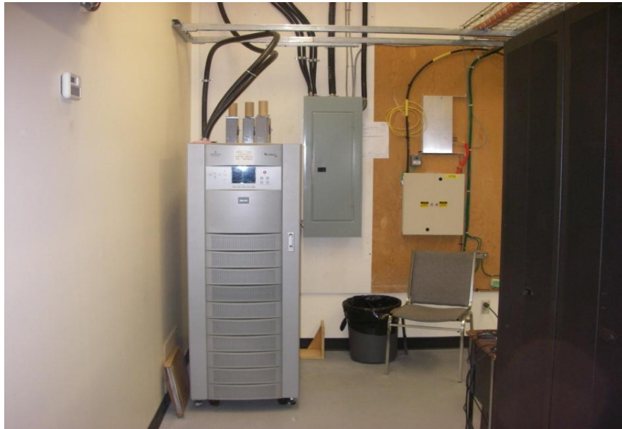
UPS - BACK UP POWER SUPPLY
