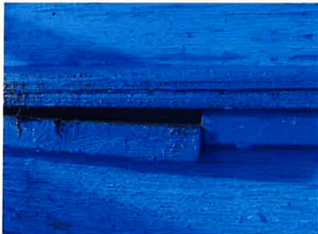
Some of the delaminating occurring throughout the bleachers with the plywood
