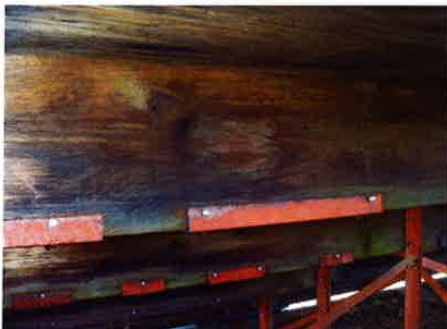
Extra supports were added but note the bolt position in the angle iron. The Engineer did not like the position as they are very close to the edge because of the addition of another layer of plywood.
