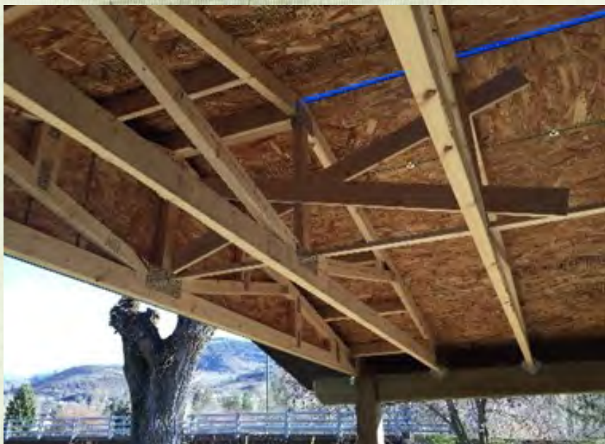
Roof Trusses with Hurricane Ties
