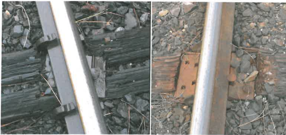
Relative size comparison of single shoulder tie plates (left) and double shoulder (right) tie plates
