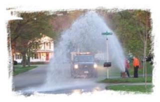
water quality in the water distribution system. The benefits include maintaining and potentially improving the water quality level in the mains. This method will also reduce bacteriological growth, restore disinfection residuals, improve color, control
